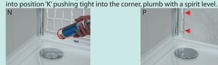
11. Apply a thin bead of waterproof sealant along the top of the Cladseal.'N'
